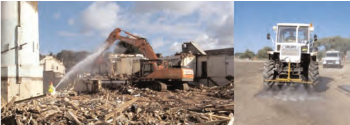
Figure 14- Control measures during demolition activity
